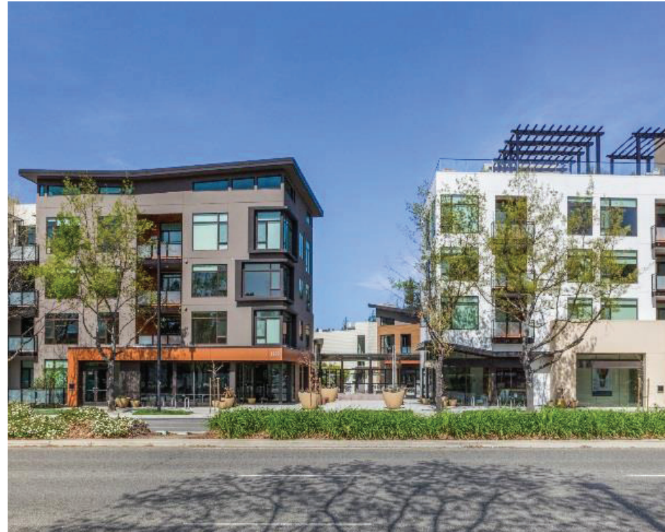
1720 W. ECR, MOUNTAIN VIEW (MONTROSE APARTMENT) - COMPLETED
