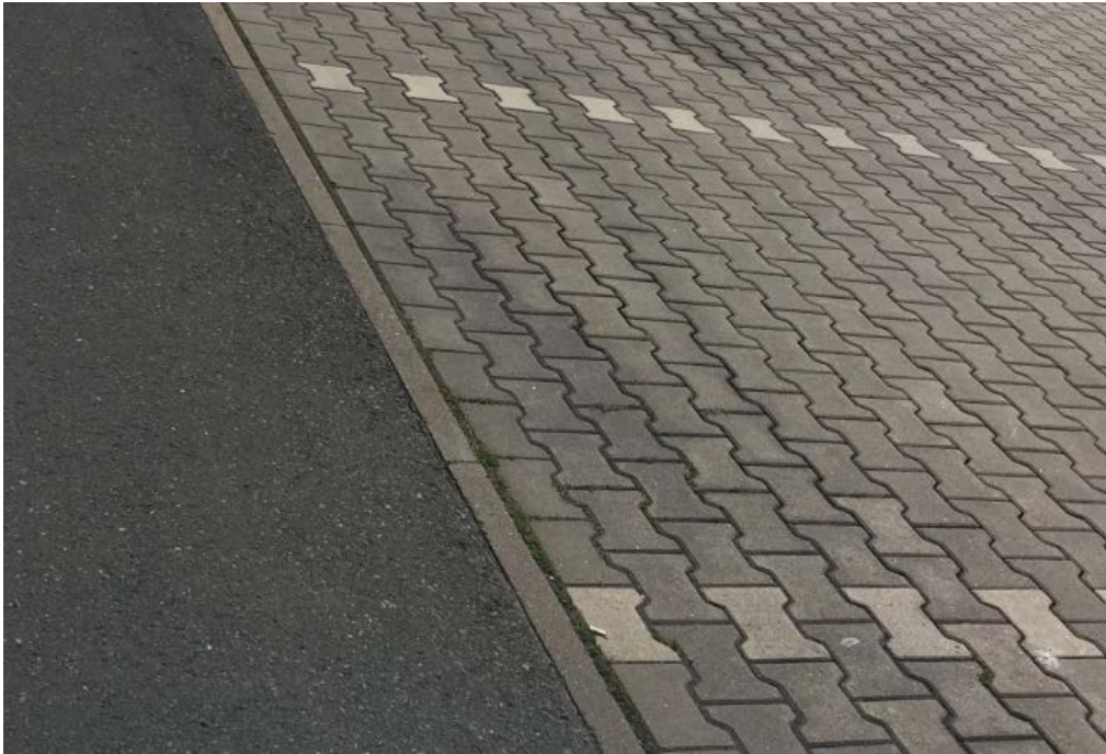
Figure 4 - Permeable concrete pavers with lateral edge confinement adjacent to road (NCE)
