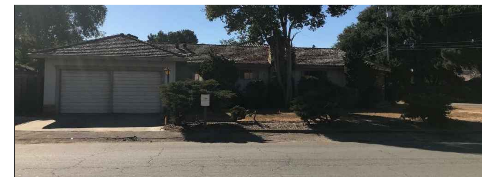
VIEW OF EXISTING FROM RICHARDSON AVE.
