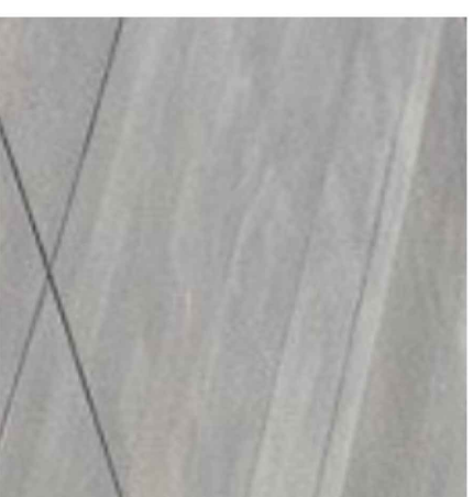
#6 Poured Gray Exterior Concrete
