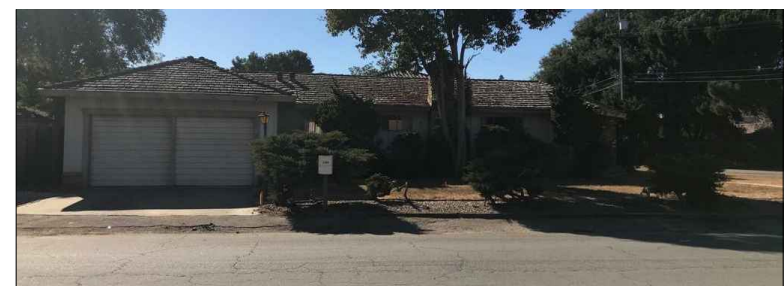
VIEW OF EXISTING FROM RICHARDSON AVE.
