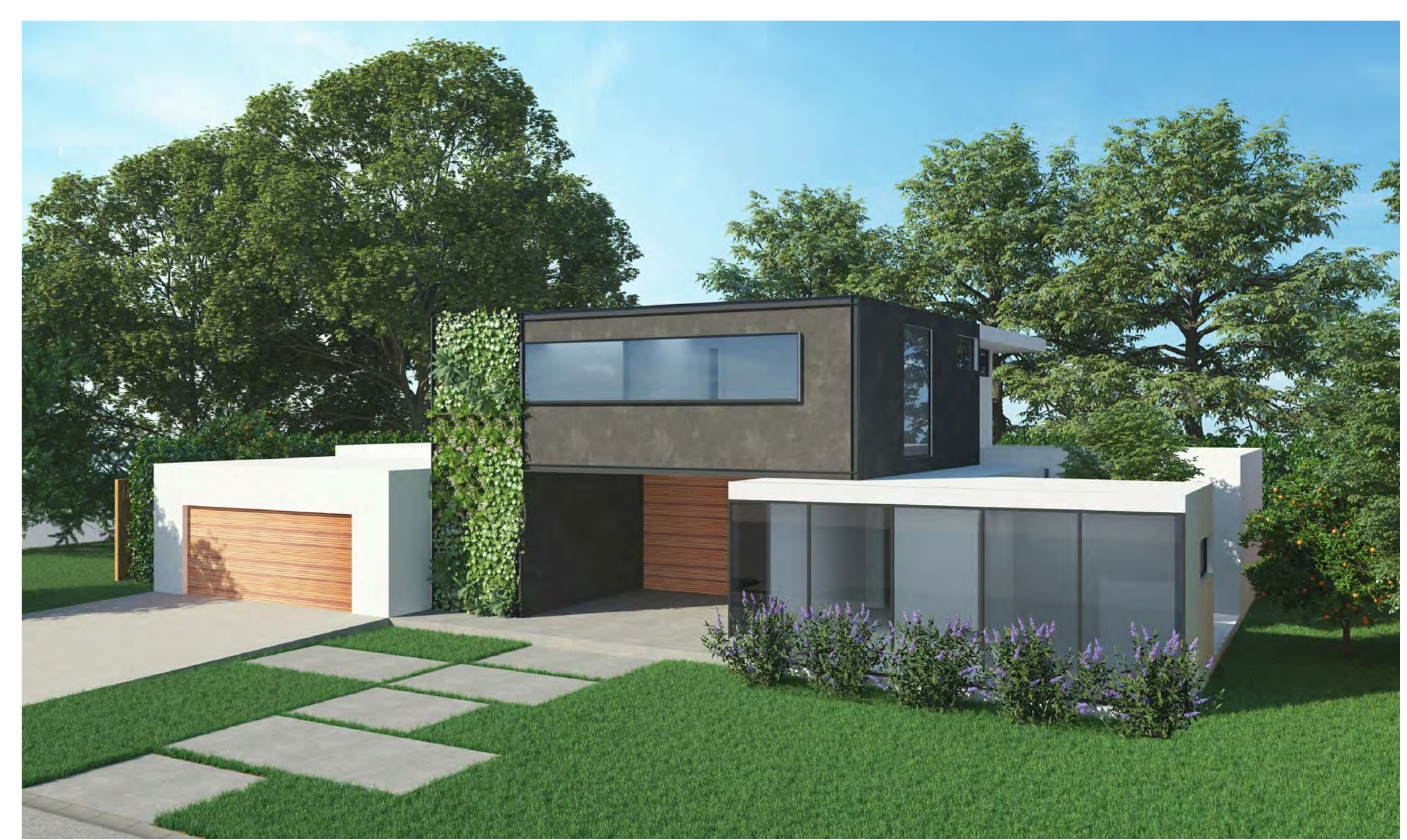
745 CAMPBELL AVE - W/O LANDSCAPING
