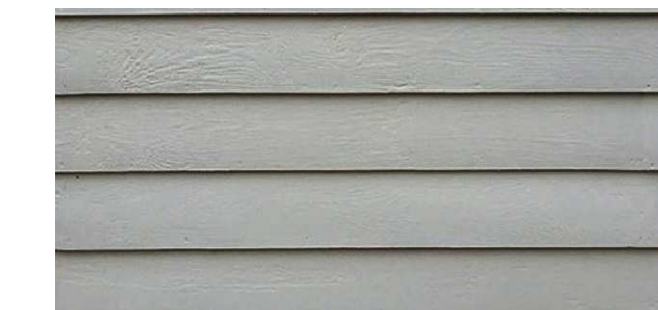
HORIZONTAL WOOD SIDING, 10" PLANK PAINTED HARDIE-PLANK LAP SIDING SHERWIN WILLIAMS: "NORTHSTAR SW 6246"
