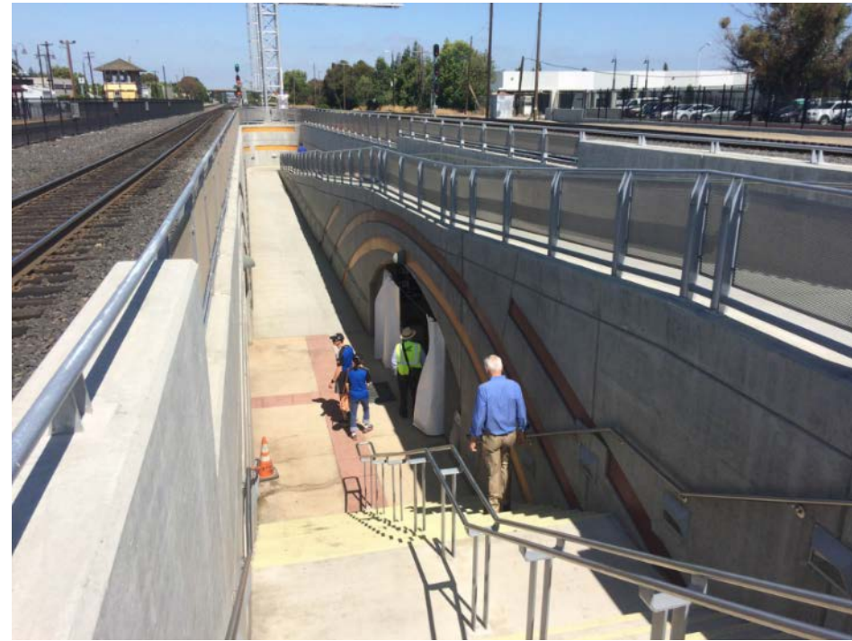
Santa Clara Pedestrian Undercrossing, opened June 2017
