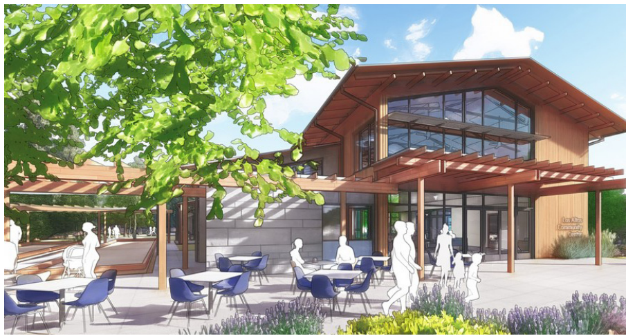
LOS ALTOS COMMUNITY CENTER (IN CONSTRUCTION) 5
