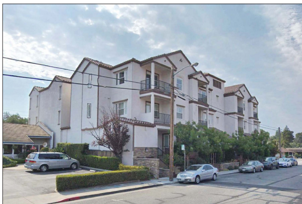
Multifamily Development across First Street
