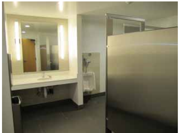
16. View of a typical restroom located inside the subject property building.
