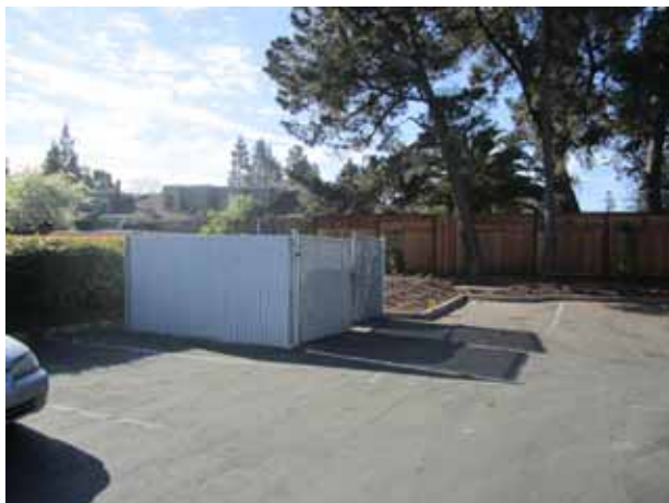
5. View of the dumpster bins enclosure located at the south-southeastern portion of the property.
