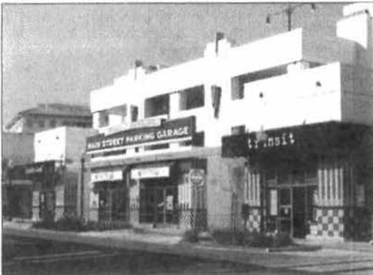
Ground level commercial uses and upper floor setbacks are techniques that relate parking structures to adjacent smaller scale development.
