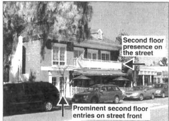
Strong presence of second floor uses on the street
