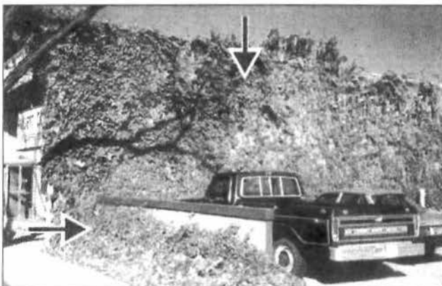
Use low walls to screen the view of cars from adjacent sidewalks and landscaping to soften blank walls.
