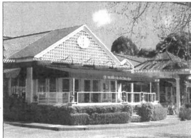
Traditional building forms, architectural details, and integrated landscaping assist in relating the parking lot frontage to an overall village scale and character.
