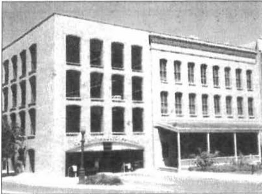
Facade materials and opening proportions help relate this parking structure to its surrounding neighbors.
