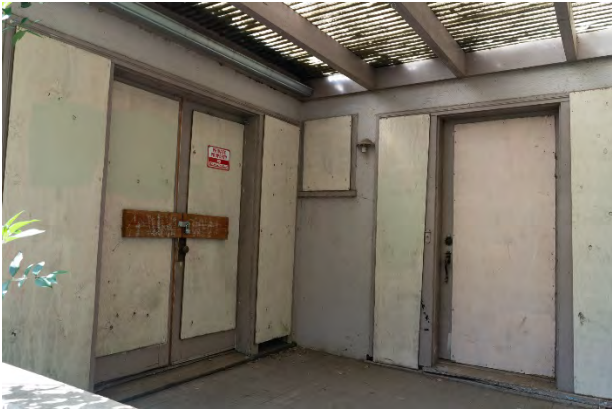
Figure 4: Entrance porch at northeast corner of building. Looking southwest.
