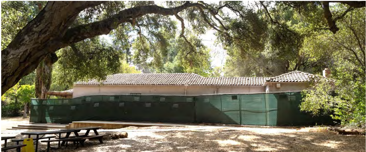
Figure 3: Primary (north) façade of the Halsey House, largely hidden by chain-link fencing. Looking slightly southeast.
