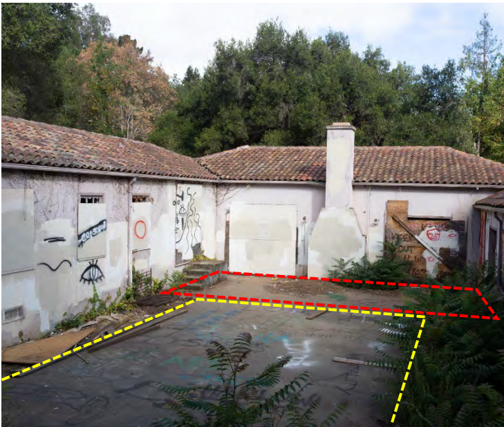
Figure 16: View of rear courtyard, looking north. Red dashed outline shows original patio. Yellow dashed outline shows area of concrete infill.
