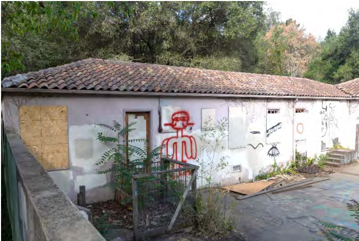
Figure 18: West side of courtyard (east-facing wall), looking northwest.
