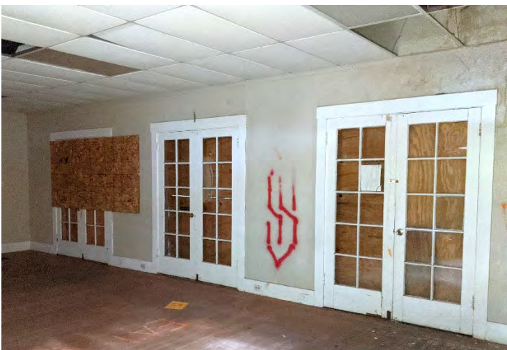
Figure 6: Interior view of French doors that open to north patio along north façade. Looking slightly northwest.
