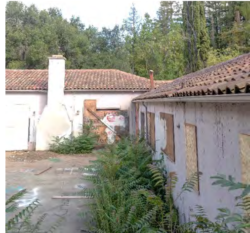
Figure 19: North and east sides of rear courtyard (south- and west-facing wall). Looking north over rear courtyard wall.
