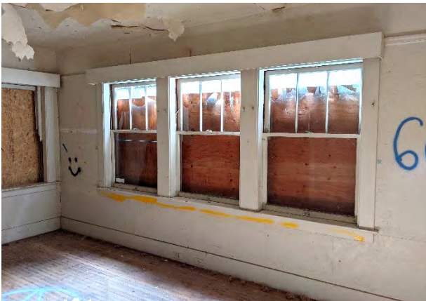
Figure 14: Interior view of three grouped typical double-hung windows along south façade of west wing. Looking southeast.
