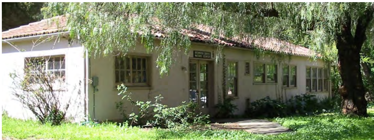
Figure 10: East façade of Halsey House in 2003. Source: City of Los Altos.
