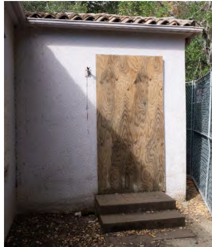
Figure 9: Secondary entrance to 1928 addition at west end of primary façade. Looking northwest.
