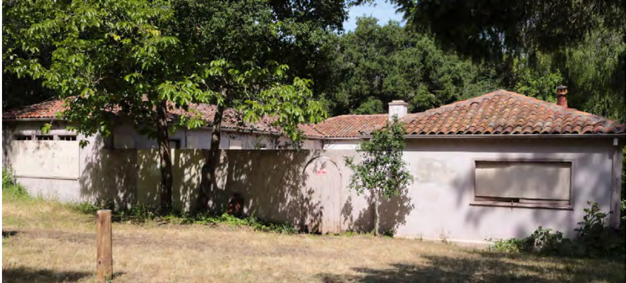
Figure 13: South façade with rear courtyard wall. Looking slightly northwest. Source: HSR by ARG, taken in May 2019.
