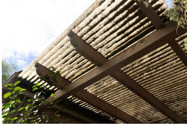
Figure 5: Wood pergola and plastic roof over entrance porch at north façade. Looking southwest.
