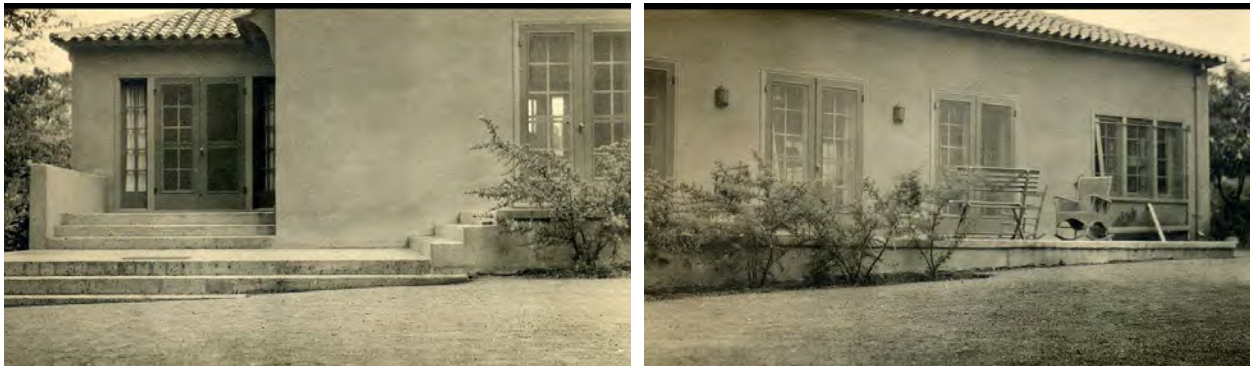
Figure 25: Two photographs of the Halsey House prior to 1928, showing the original full length of the primary (north) façade which ended just west of the three grouped eight-lite casement windows. Source: Los Altos History Museum Collections, courtesy of Katherine Halsey Buss.
