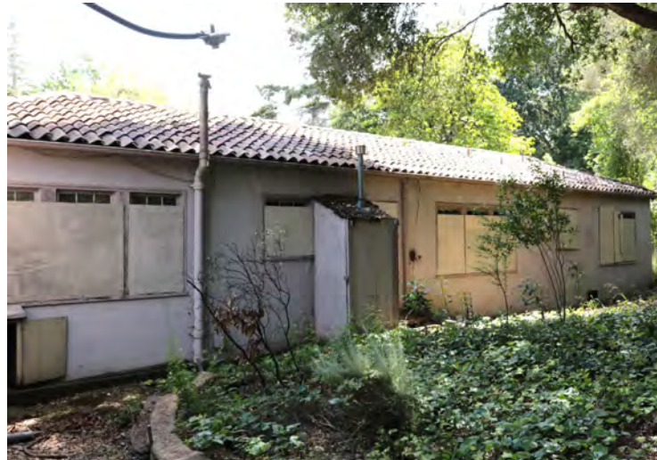
Figure 12: West façade of original section of residence. Looking slightly southeast. Source: Halsey House HSR by ARG, taken in May 2019.
