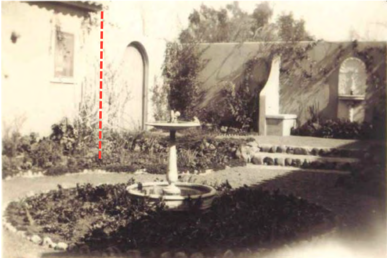
Figure 26: Historic photograph of the courtyard in the late 1920s or early 1930s, showing the original configuration of the east wing and the courtyard wall. The red dashed line indicates the original end of the east wing prior to the construction of an addition at an unknown date likely in the 1930s. Today the round-arched courtyard door is located in the south wall, just left of the bench in this photograph. Source: Los Altos History Museum Collections. Edited by Page & Turnbull.
