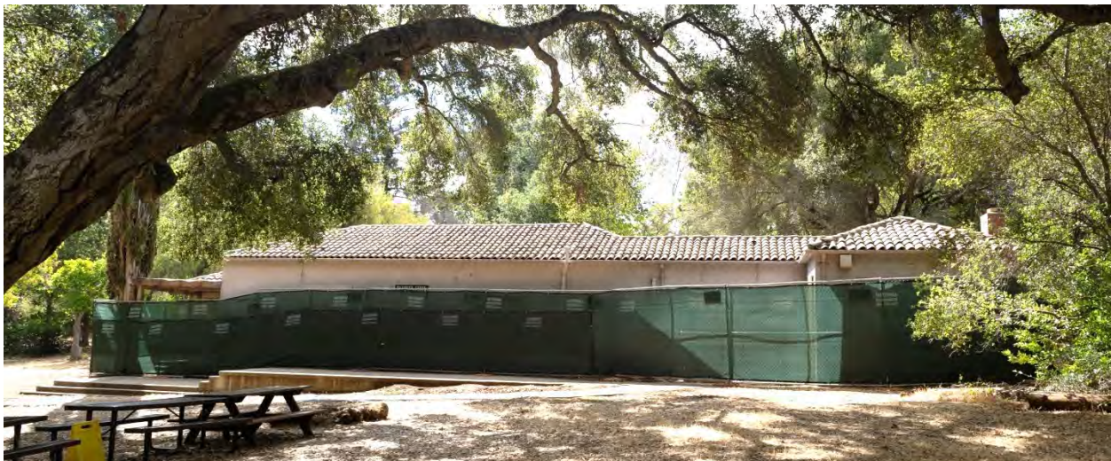
Figure 3: Primary (north) façade of the Halsey House, largely hidden by chain-link fencing. Looking slightly southeast.
