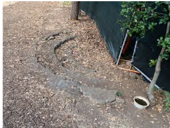
Figure 15: Semi-circular steps to gate in south façade of courtyard wall. Looking down and slightly northwest.
