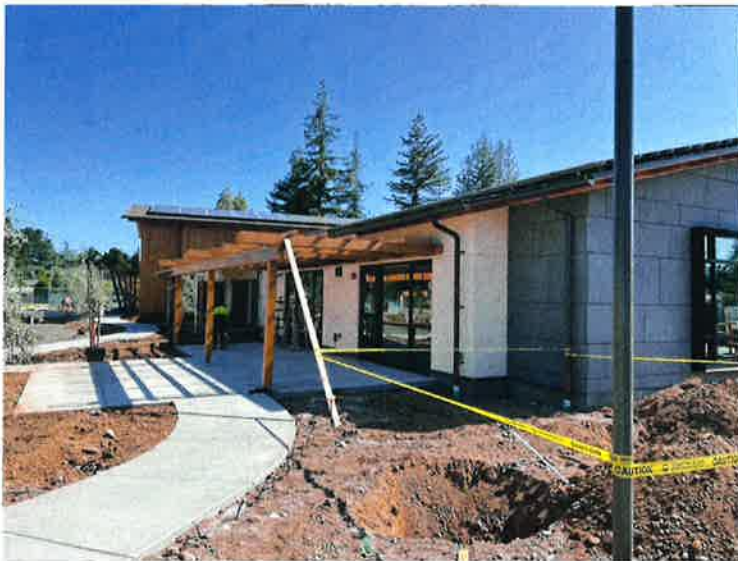
Exterior Progress at Senior Room
