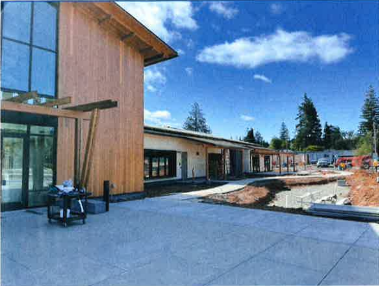
Exterior Progress at Main Entrance
