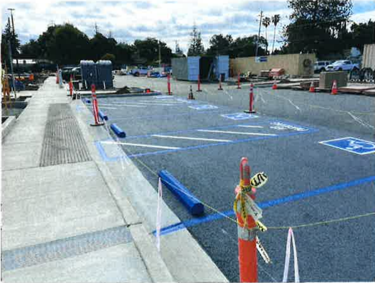
Striping in Parking Lot
