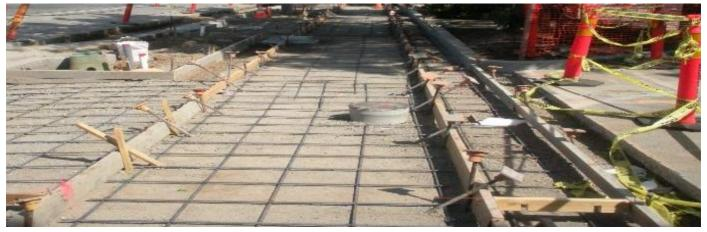
The annual concrete sidewalk and curb/gutter repair project is intended to address the highest priority repair locations. The primary focus is on the replacement of damaged sidewalks that represent hazards to pedestrians. Staff continually receive complaints from residents regarding cracks or uplifted sidewalks that could cause a "trip and fall" type accident.
