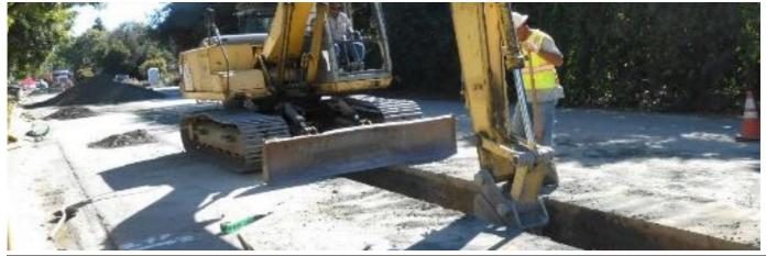
The 2013 Sanitary Sewer Master Plan Update recommended replacement of segments of pipes located at various locations throughout the City that are included in the 30-day focused cleaning schedule that have severe sags. Such sags can cause accumulation of debris and grease which necessitates frequent cleaning.
