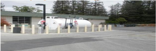
The fuel dispensing island at the Municipal Services Center (MSC) has an above ground holding tank with containment wall around it. It is necessary to build a canopy to limit storm water entering the contained area and to provide cover for the fueling station to prevent excessive weathering of the electronic screens and keypads.
