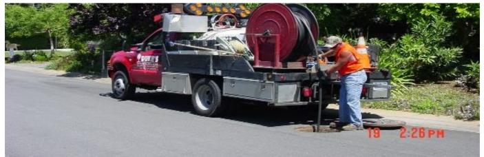
The Sewer Master Plan Update recommends that an annual project be performed to chemically remove invasive tree roots within sewer mains. Chemical root removal products currently on the market provide protection from future root growth for two to three years following application.
