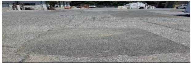
The pavement at the City's Municipal Services Center (MSC) is deteriorating and in need of repair. This project will include the design and construction of pavement rehabilitation and improvement of the current drainage system. The design will also incorporate the green infrastructure features into the project to comply with the current stormwater permit requirements.
