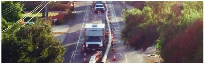
This project consists of work to repair pipe corrosion using the cured-in-place pipe (CIPP) repair method for the trunk sewer. The pipe sizes range from 24-inches to 42-inches, which are the largest pipe diameter sections in the system that deliver sewage to the Palo Alto Regional Water Quality Control Plant. The trunk sewer rehabilitation is prioritized to rehabilitate the reaches that are most corroded as determined from inspections of the trunk sewer pipe.
