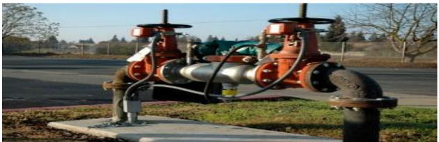
The project will install backflow preventers for all City-metered water connections. The Cross Connection Control Program is designed to meet the requirements of the California Code of Regulations, Title 17, Public Health Sections 7583 through 7605. Failure to install and maintain such devices may lead to a water service interruption and possible loss of water services.
