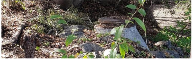
This project scope includes replacing, and for some segments realigning, 53 sewer main segments, located along or near Adobe Creek. This compromises a total of 6,580 linear feet of pipe replacement. The existing 6-inch and 8-inch pipes will be replaced with new 8-inch pipe to increase capacity. The sewer line segments identified for this project are located near the City's border with the Town of Los Altos Hills, north of Manresa Avenue and south of Edith Avenue.
