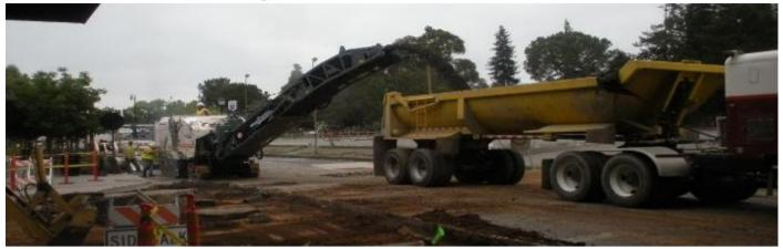
The annual street resurfacing project places an overlay of asphalt concrete (AC) on existing street surfaces approaching the end of their useful life, as evidenced by cracking and minor pavement failures. Installation of pavement fabric, striping, repair of damaged curb and gutter, and minor drainage improvements are also included in this project where necessary.
