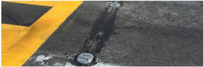
The City has existing pedestrian-activated in-pavement warning light systems in and around Downtown. The existing systems are past their useful life and failures in the equipment are starting to occur. This project will replace failed in-pavement lights and adjacent signs with flashing lights at the following locations:
