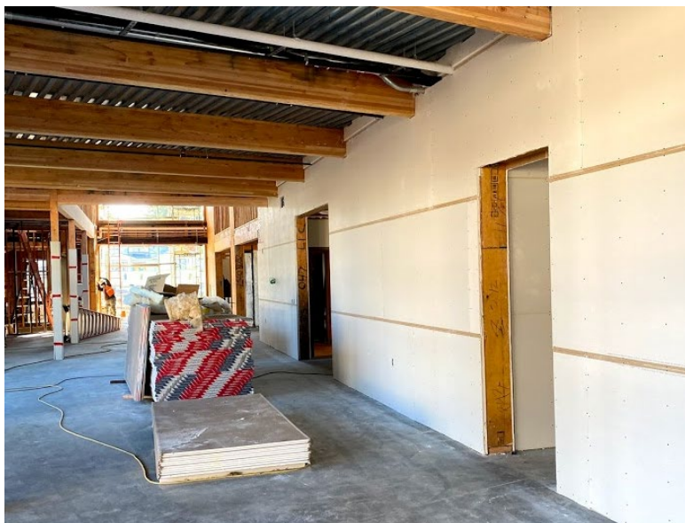
Interior Progress at South Lobby
