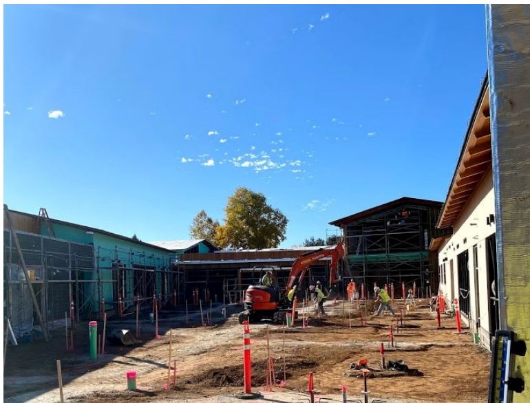
Exterior at Main Courtyard
