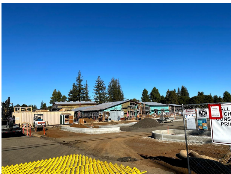
Exterior Progress along Hillview Ave.
