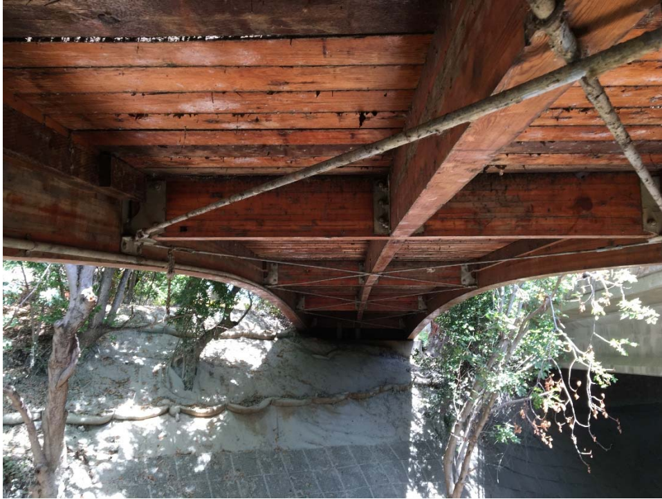
Figure 3 - Pedestrian Bridge soffit looking east, with bracing and attached utility line
