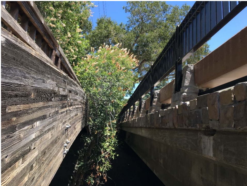
Figure 6 - South side of Pedestrian Bridge with close proximity to vehicular bridge
