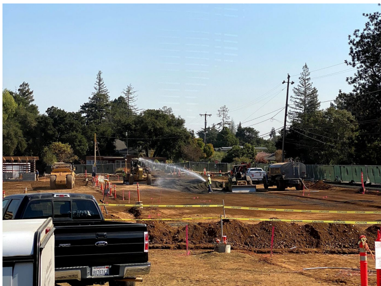
Grading Operation at Hillview Parking Lot
