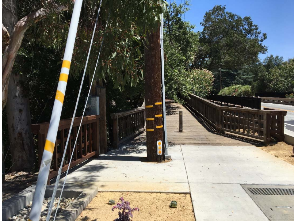
Figure 1 - Pedestrian Bridge looking east with close proximity to utilities
