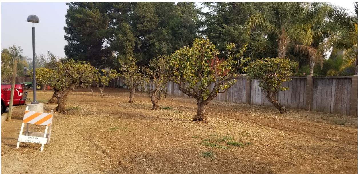
Figure 3: Looking north from construction area, the Apricot trees outside the construction area are visible.
