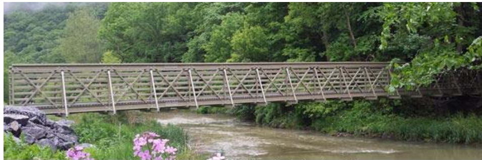
Hiking Trail Bridge – 85' x 4' located in Loysburg, PA
