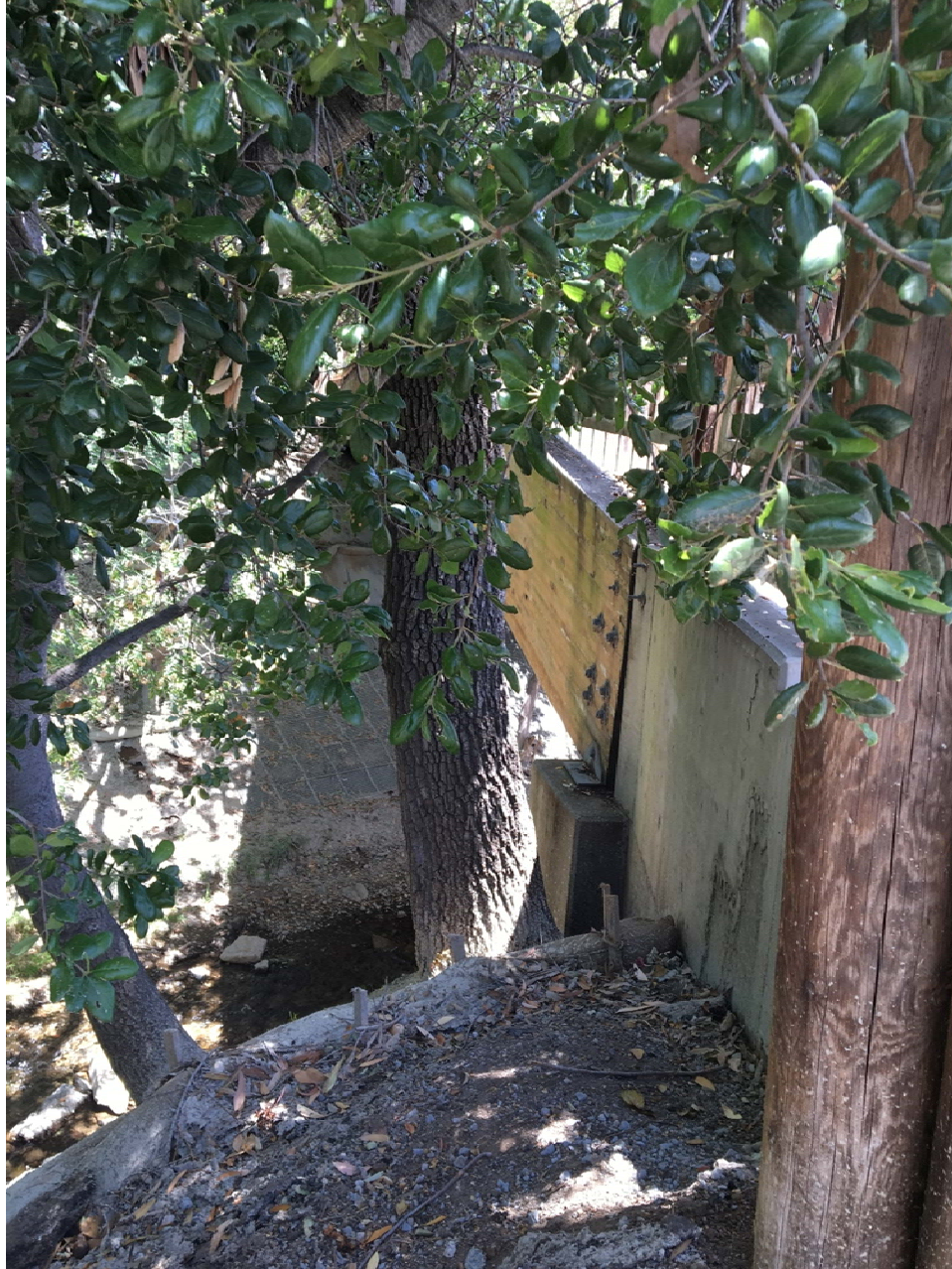
Figure 7 - Northwest corner of Pedestrian Bridge with close proximity to existing trees and utility pole
