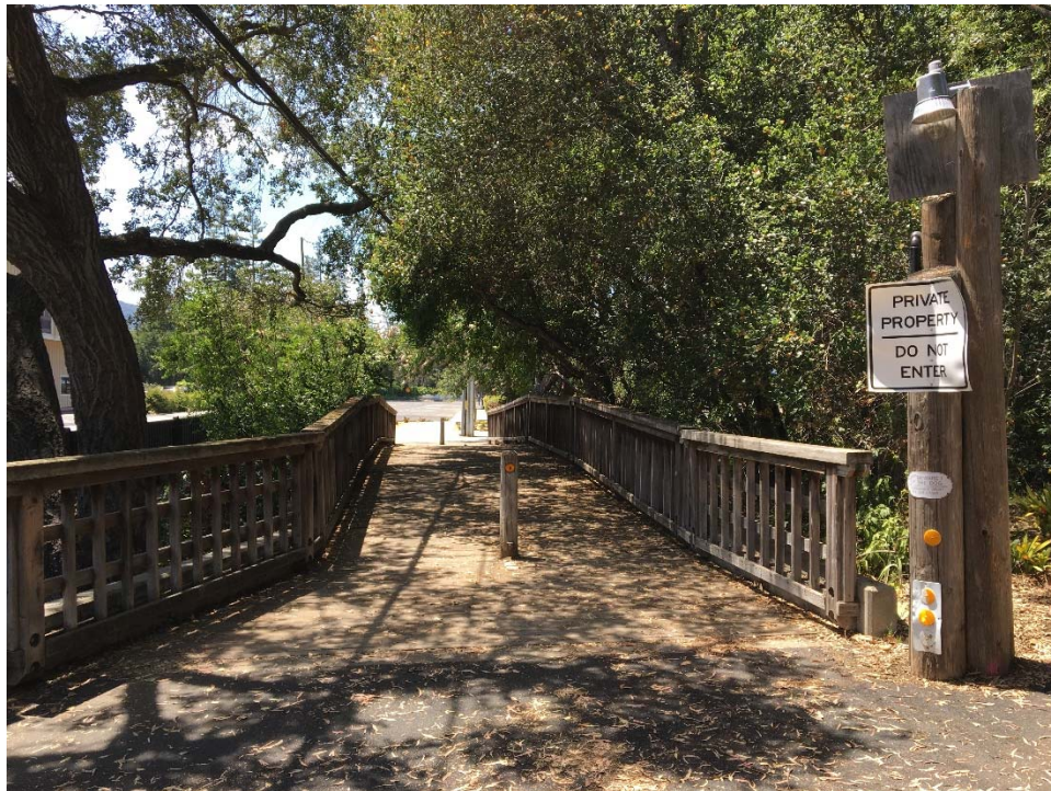
Figure 2 - Pedestrian Bridge looking west with close proximity to trees and overhead utility
