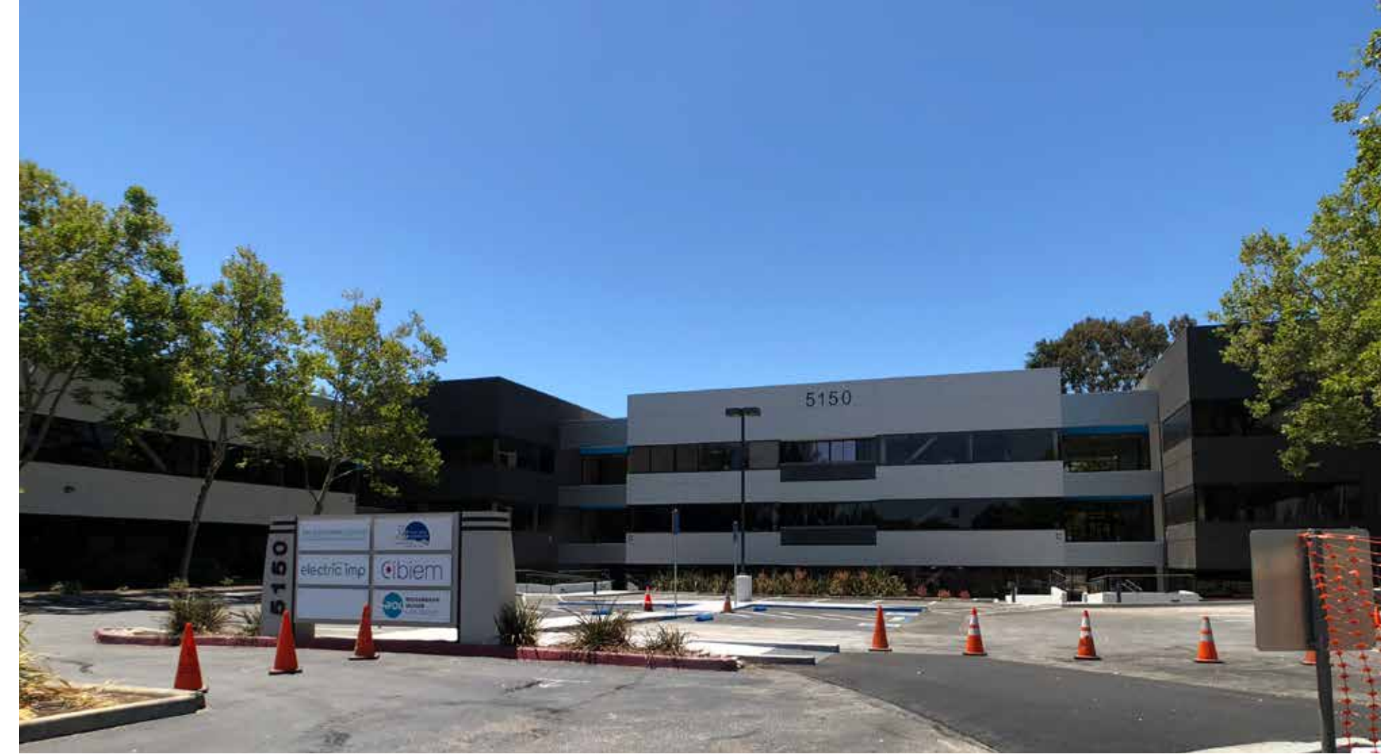
2. VIEW OF EXISTING BUILDINGS AT RENGSTORFF AVE. TERMINUS
