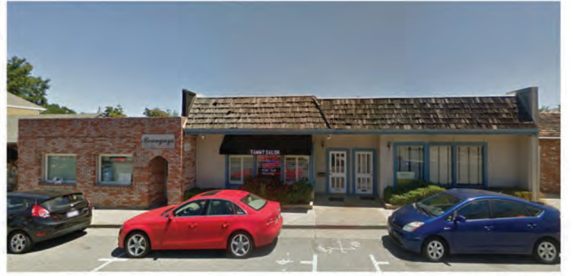
389 FIRST STREET - EXISTING SITE
