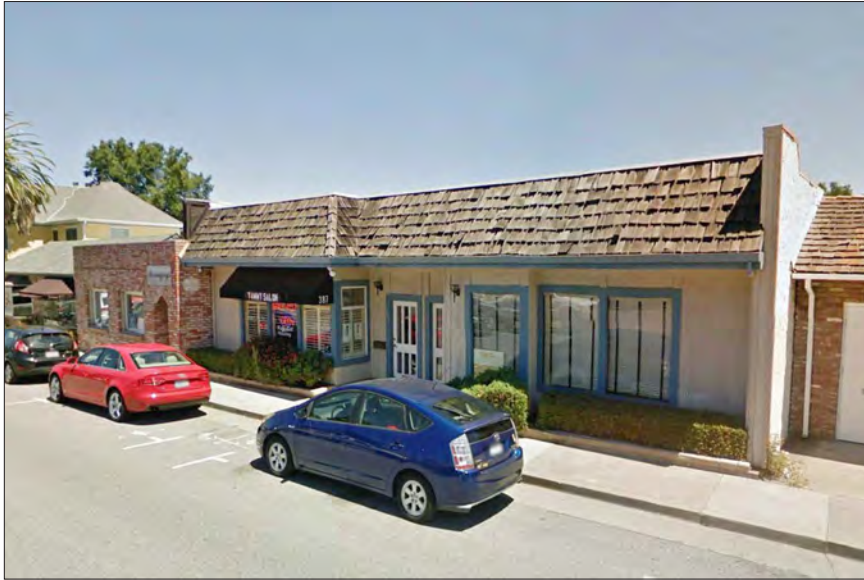
The Site and Existing Buildings
