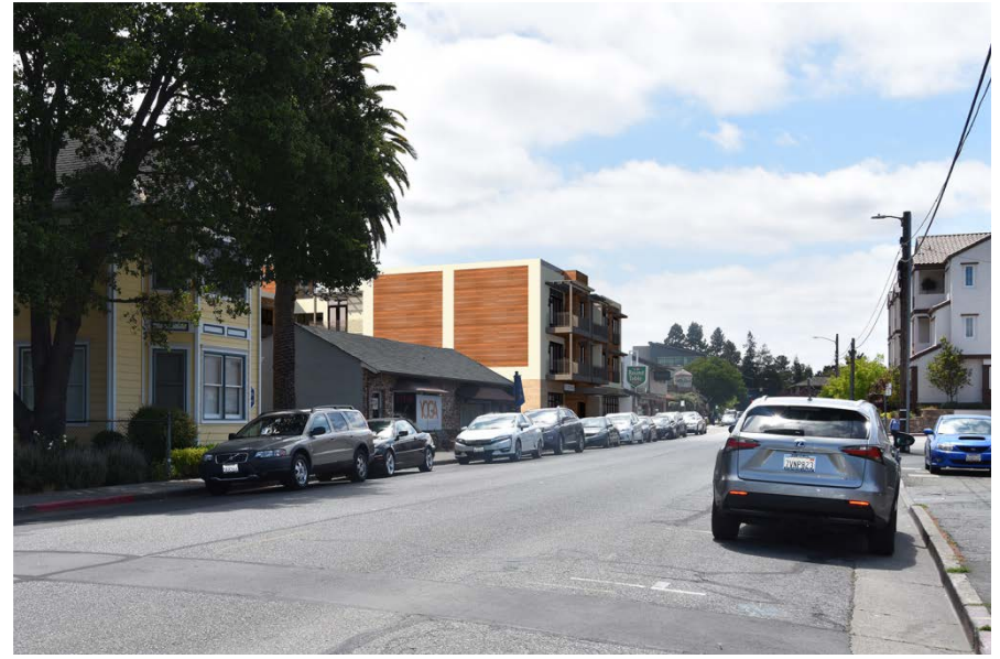
VIEW FROM FIRST STREET & WHITNEY STREET
