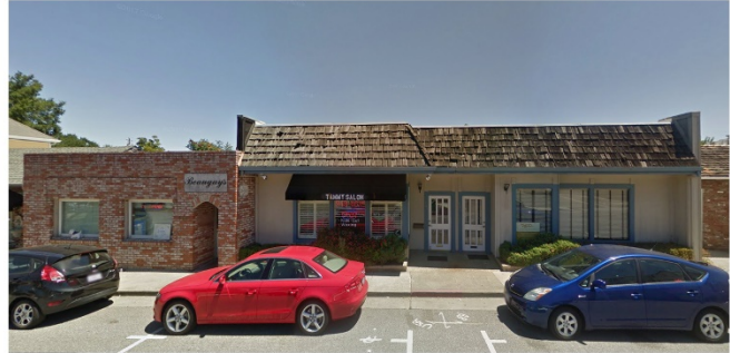
389 FIRST STREET - EXISTING SITE
