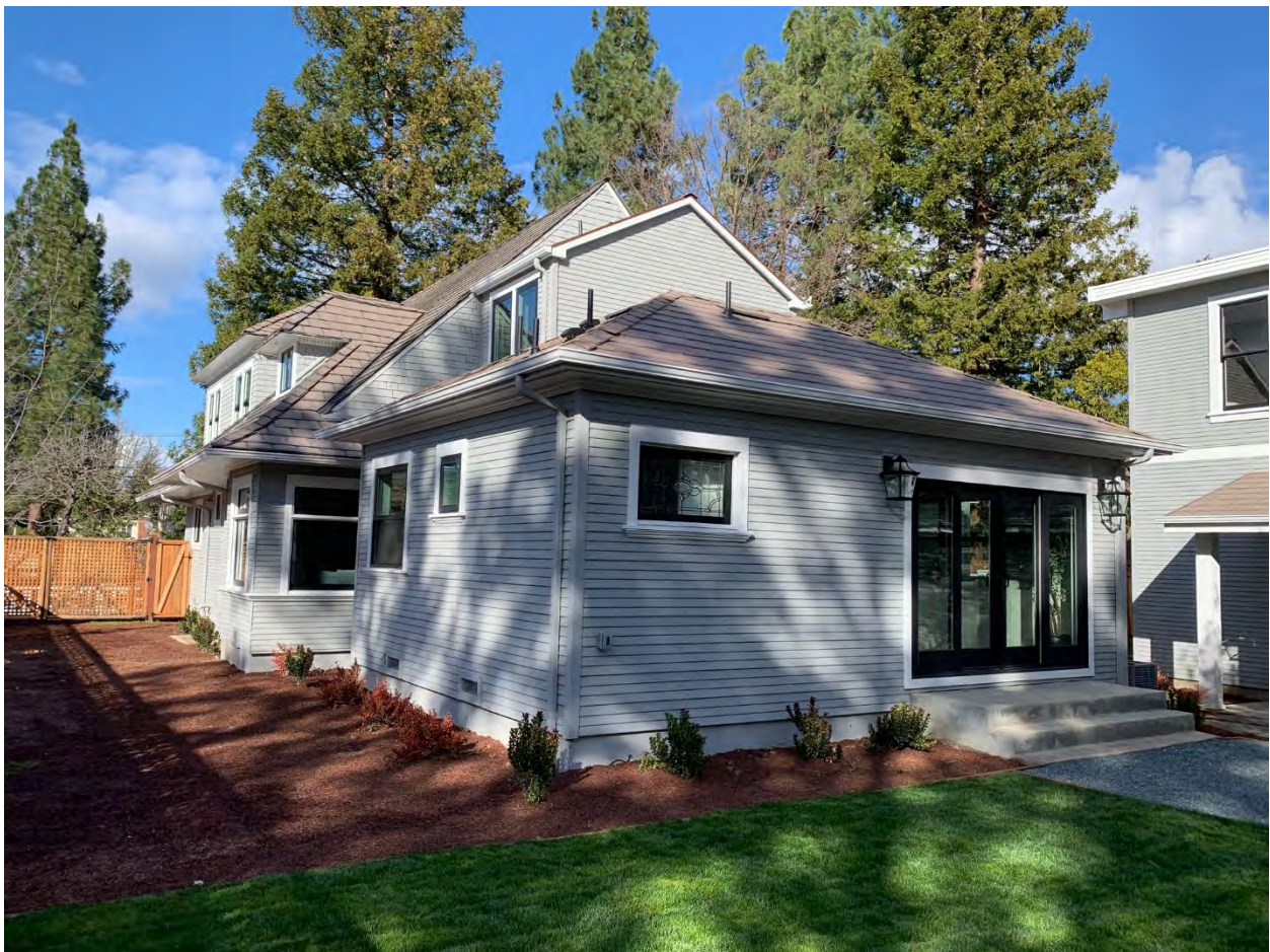
Photograph 4 A (Below) View: Rear façade showing new addition. Date: February 17, 2019
