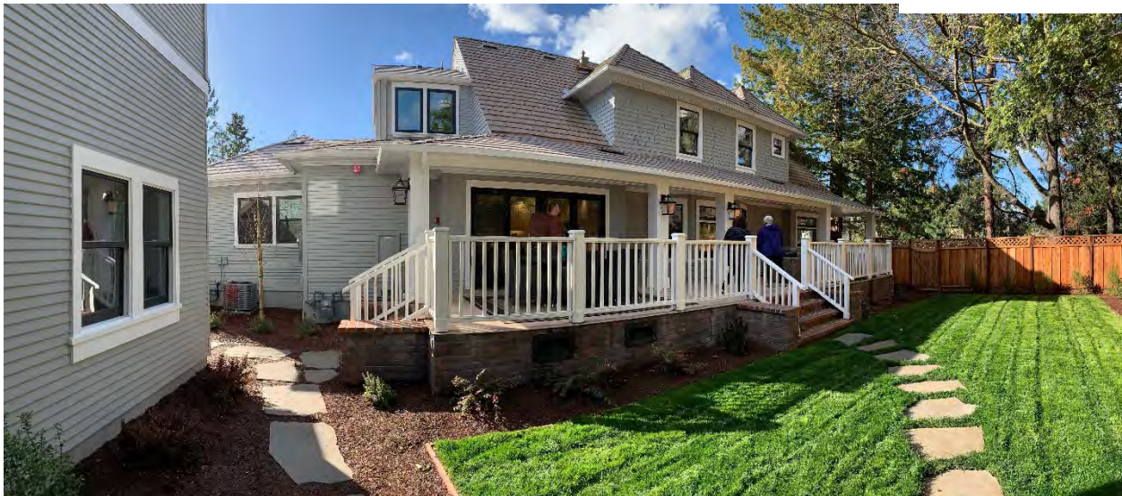
Photograph 7A 980 Covington Rd- Main house View: East façade (former south façade). Brick veneer of the extended porch and stairs reminiscent of the former addition. Vertical post railing that is code compliant height and is a style appropriate to the building. Date: February 17, 2019 Camera facing NE
