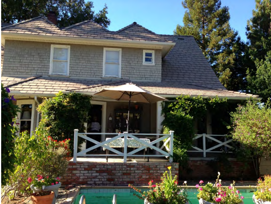
Photograph 7 View: South facade showing the additional stair landing in used brick and the western cross-brace porch railings. Swimming pool is in the foreground. Date: August, 2013 Camera facing North
