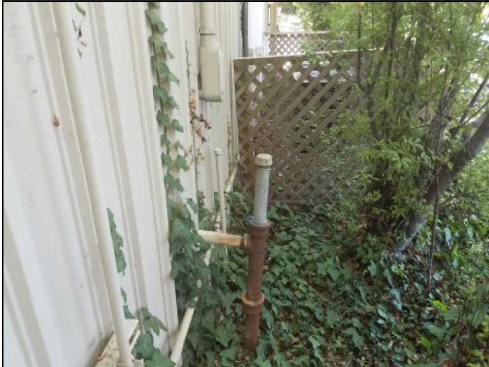
Unidentified pipe on the north side of the theater building.
