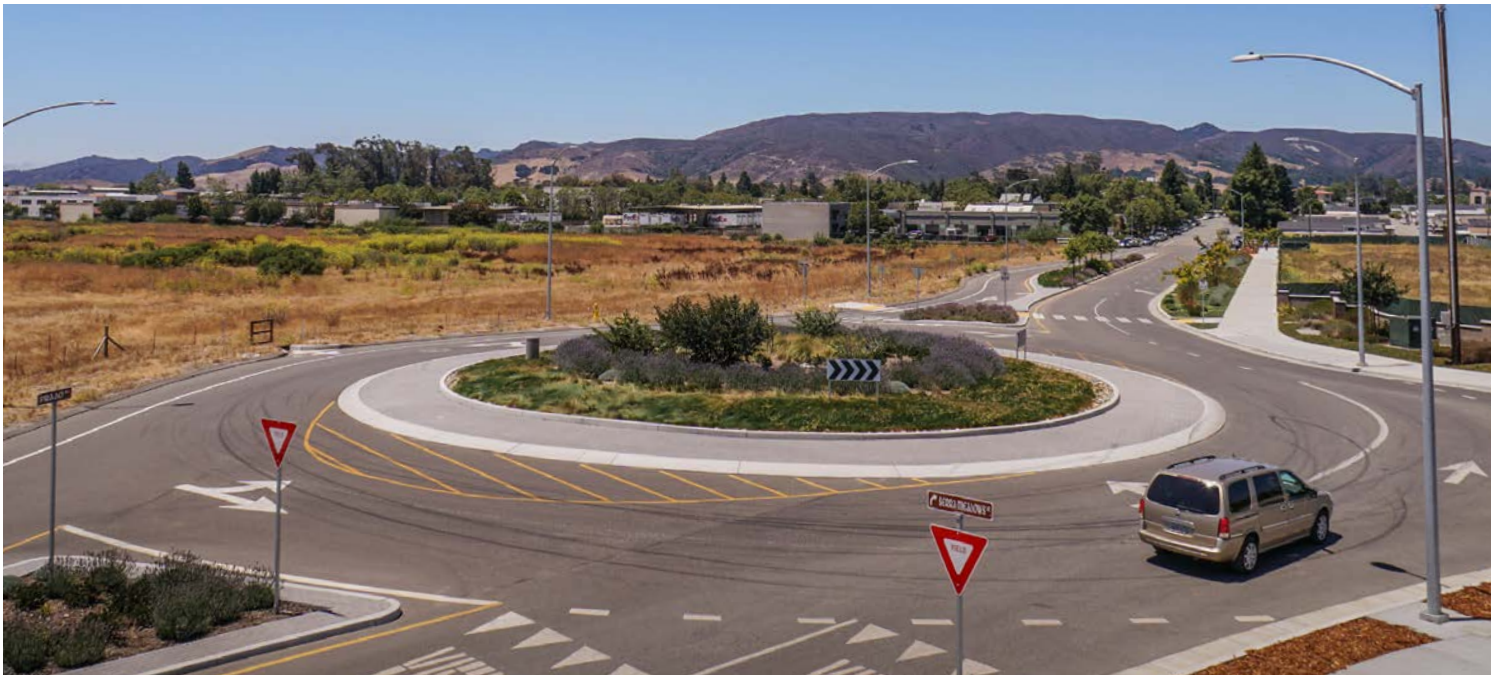
Example of a roundabout with native landscaping and accent paving at center.
