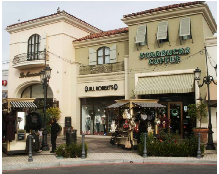
Building design should ensure flexibility to be able to adapt to changing market demands.
