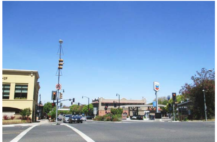
Existing Primary Entry to Downtown at Main Street and the Foothill Expressway intersection.
