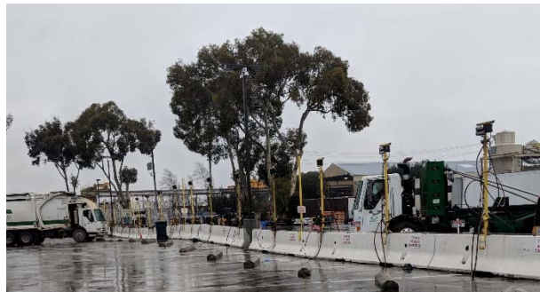
Photo #2: MTWS CNG fueling station
