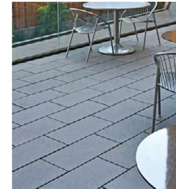
Concrete Pedestal Pavers
