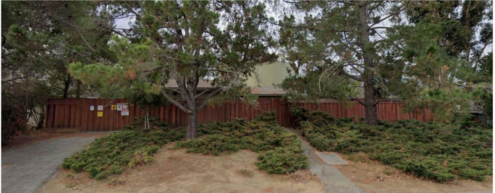
View of Station 19 from Highlands Circle
