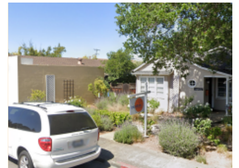
⑥ View of the single family residence on the project site at 371 First St.
