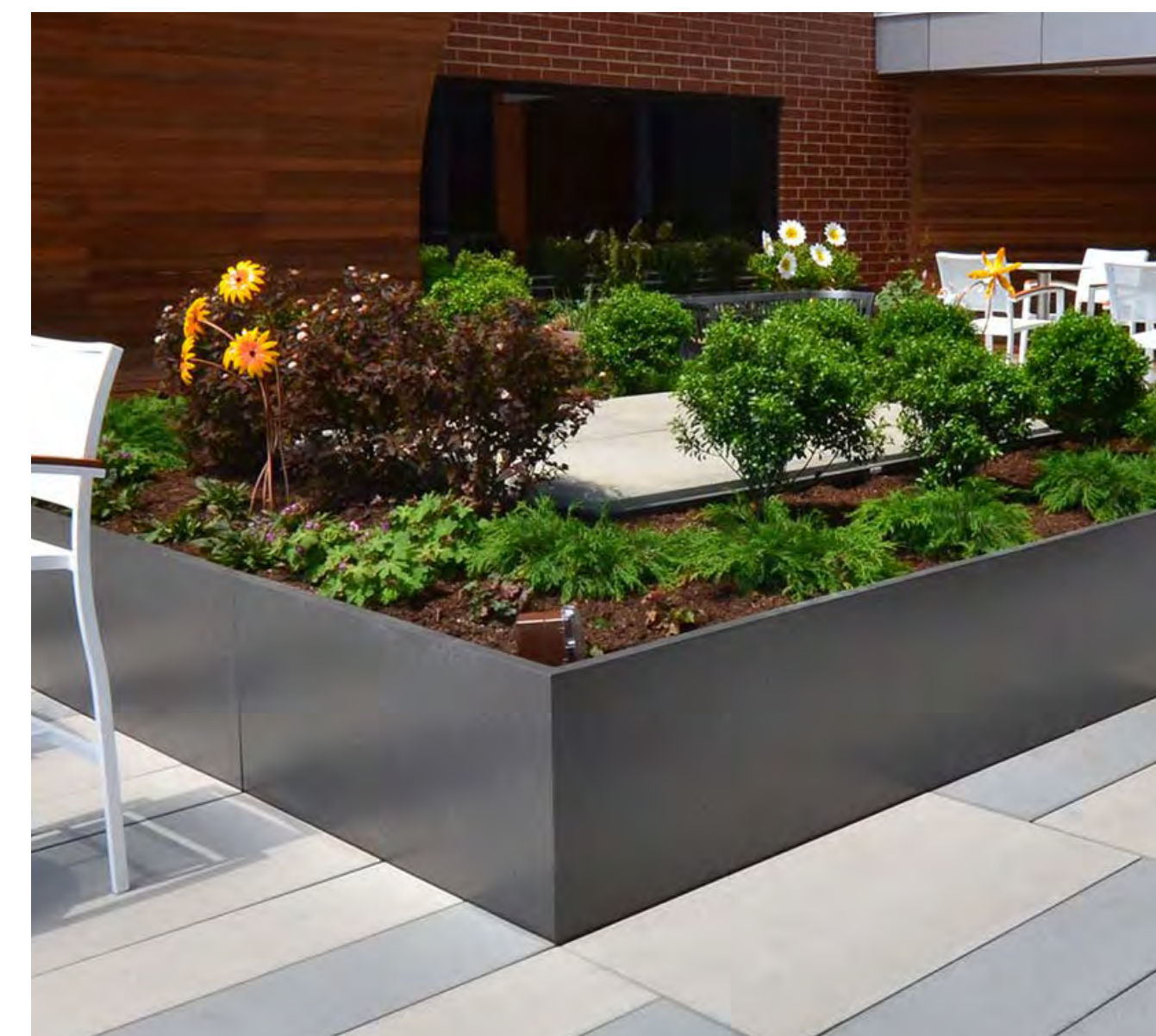
PRECAST PLANTERS - ROOF DECK
