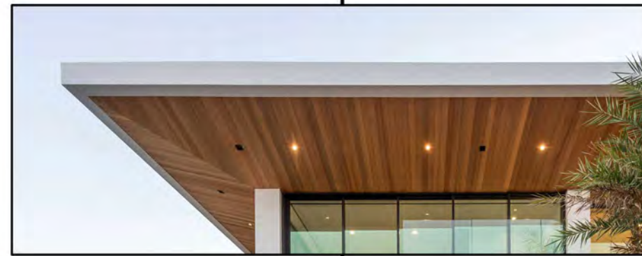
WOOD-LOOK BOARD SOFFIT AT UPPER ROOF OVERHANG
