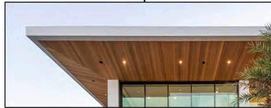
WOOD-LOOK BOARD SOFFIT AT UPPER ROOF OVERHANG
