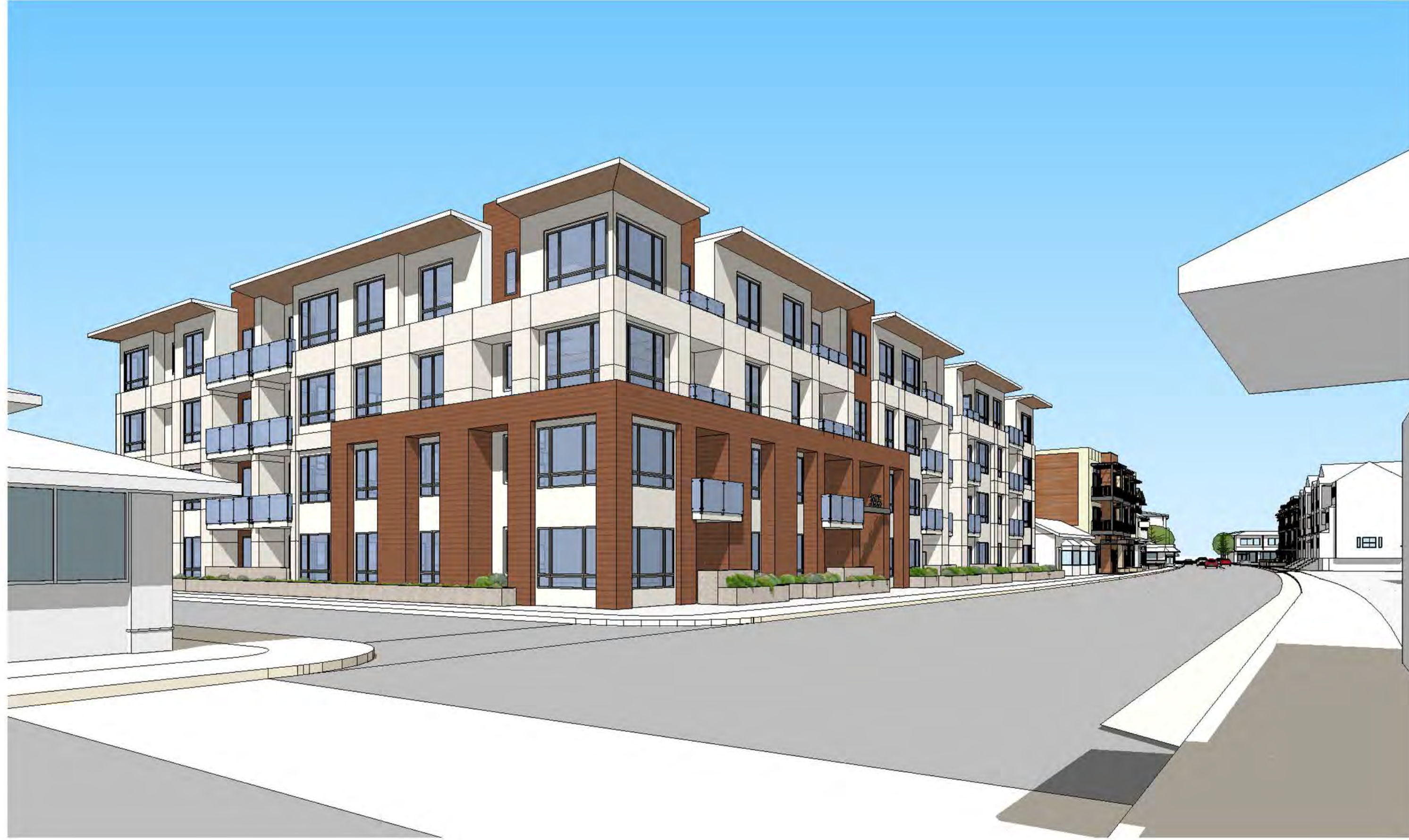
VIEW FROM WHITNEY STREET AND 1ST STREET
