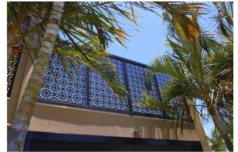
LASER-CUT STEEL SCREEN FOR BALCONY RAILING WILL PROVIDE PRIVACY WHILE ALLOWING LIGHT AND SHADOW TO PENETRATE. THE SCREENS WILL ALSO PROVIDE AN ARTISTIC ELEMENT TO THE DOWNTOWN FABRIC.
