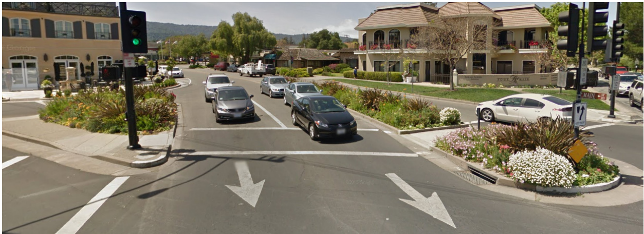
Figure 3-18: Two types of medians—slip lane and center—shorten crossing distances and create a gateway at the skewed intersection of Main Street and San Antonio Road. (Image: Google)
