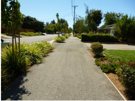
Figure 3-9: Twelve-foot multi-use path on Rosita Avenue
