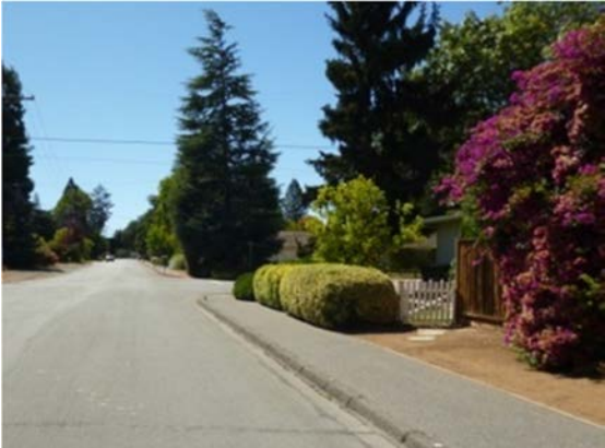
Figure 3-11: Paved shoulders often double as parking lanes, sidewalks, and bicycle facilities in many residential neighborhoods in Los Altos(left). An asphalt berm (right) converts a paved shoulder into an informal walkway.
