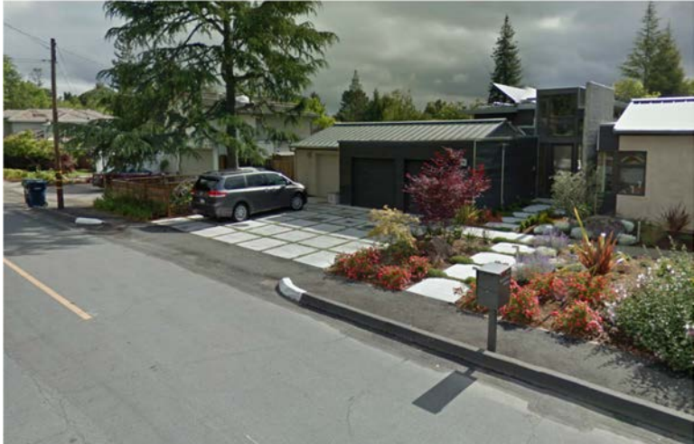
Clark Avenue Asphalt Berm-Separated Walkway Los Altos, CA
