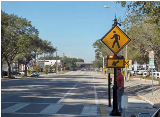
Figure 5-7: Rectangular rapid flashing beacon
