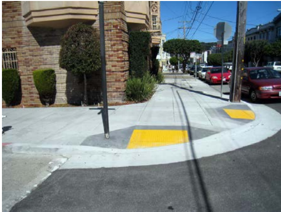
Figure 5-9: Perpendicular curb ramp in San Francisco, CA
