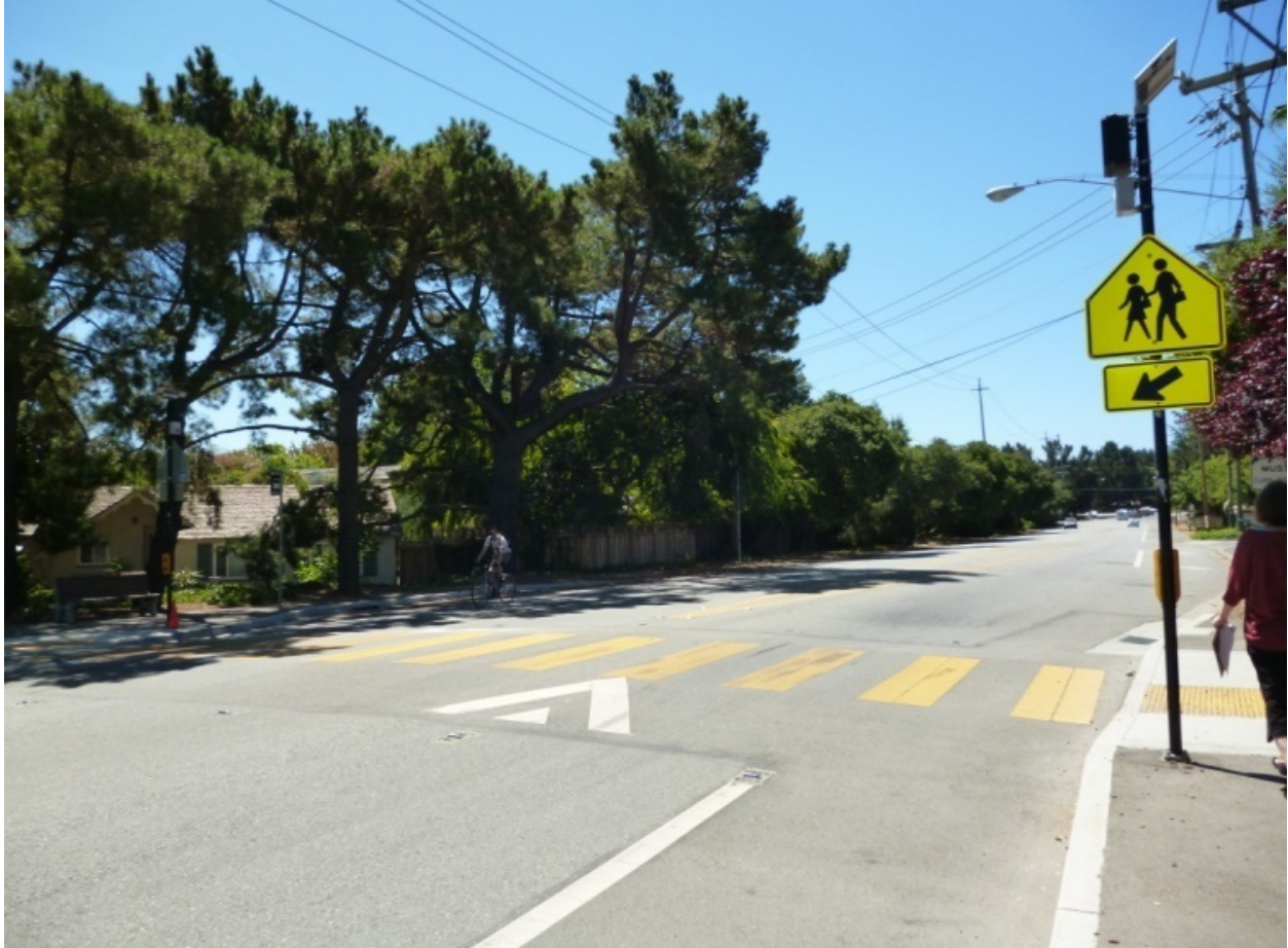
Figure 3-14: A crossing on Grant Road at Morton Avenue includes a raised crosswalk, high-visibility striping, and pedestrian-activated in-pavement flashing lights. St. Simon Elementary School is located on the west side of the crossing. A VTA Route 51 bus stop is to the east.
