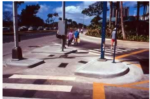
Figure 5-10: Slip lane refuge island
