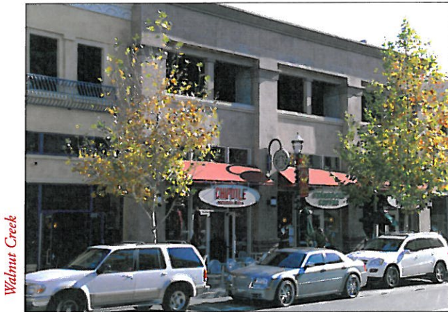
This parking structure has been designed with pilasters, and with varied facade depths, and details to relate to the module and style of nearby retail shops.
