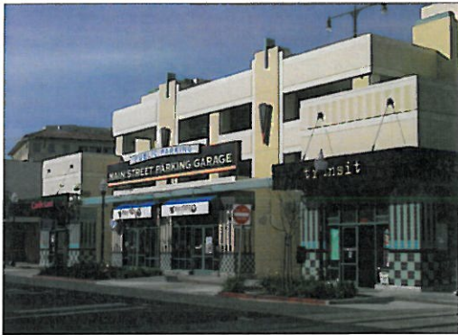
Ground level commercial uses and upper floor set-backs are techniques that relate parking structures to adjacent smaller scale development.
