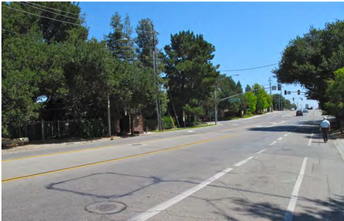
Homestead Road was one of many streets assessed for closing the gap in the Stevens Creek Trail.
